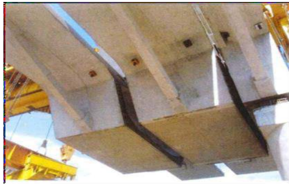
( Fig 28. Placing of segment in order)
