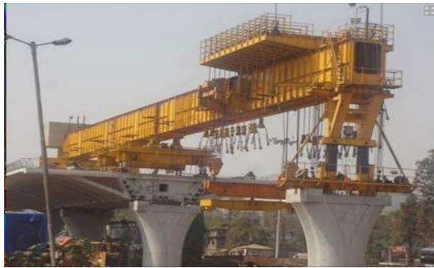
( Fig 27. Segment being lifted ad placed)
