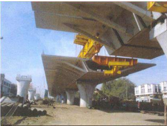
(Fig 29. Segment being placed in position)
